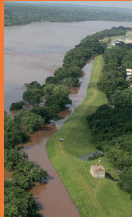
Tulsa Levee in 2019 Flood
