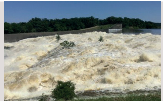
Figure 2 - Wister Lake Spillway within the Tulsa District.
