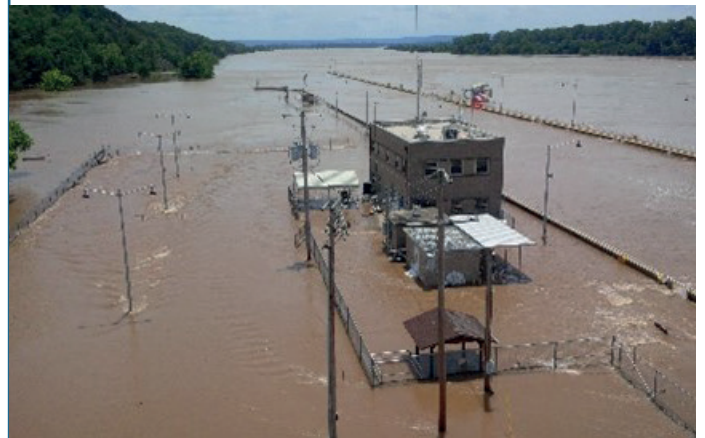
Figure 8 - MKARNS during a flooding event
